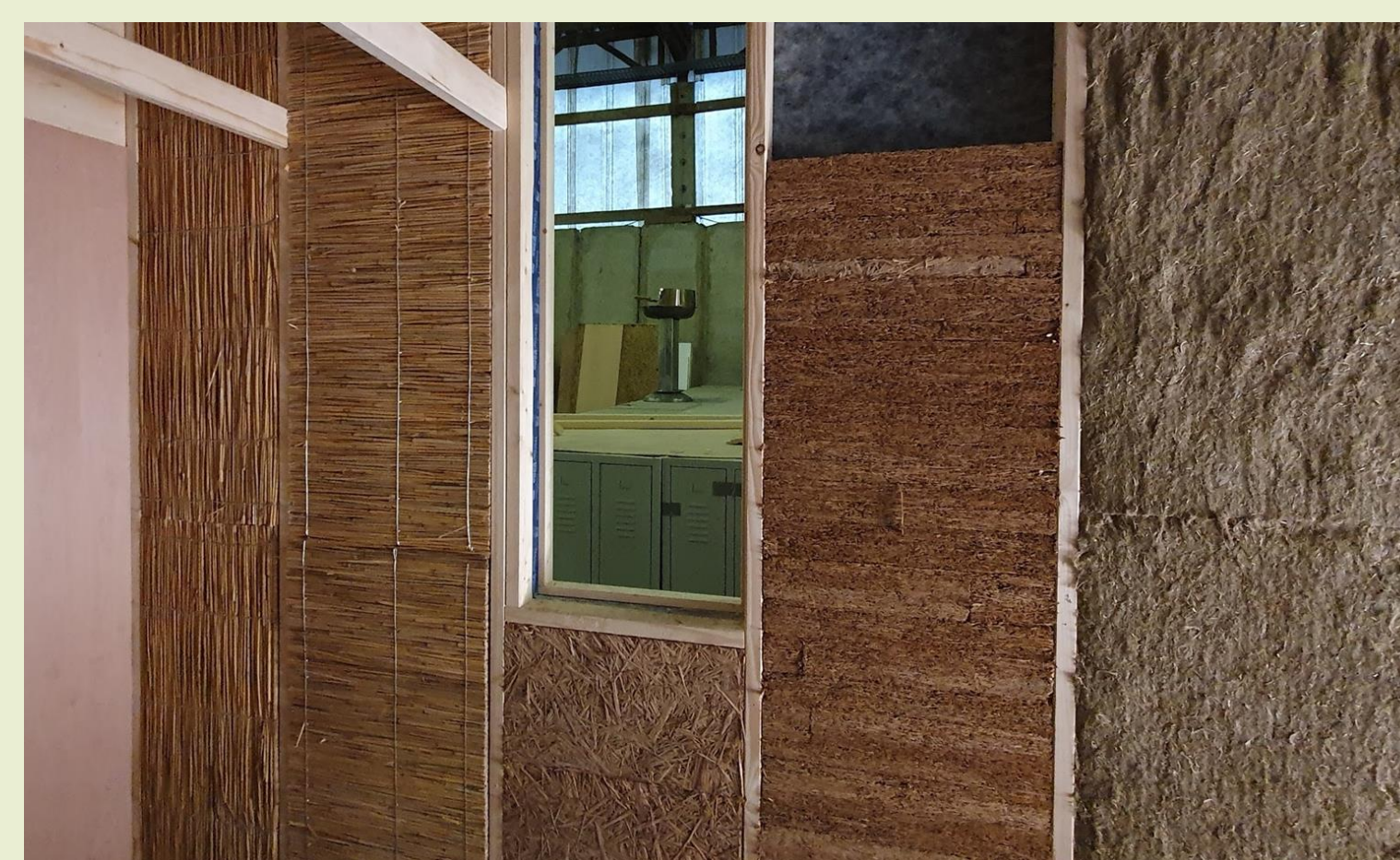
Fig. 2: paludi-insulation materials in frame construction: reed (left), cattail boards (middle), grass fibres (right).
