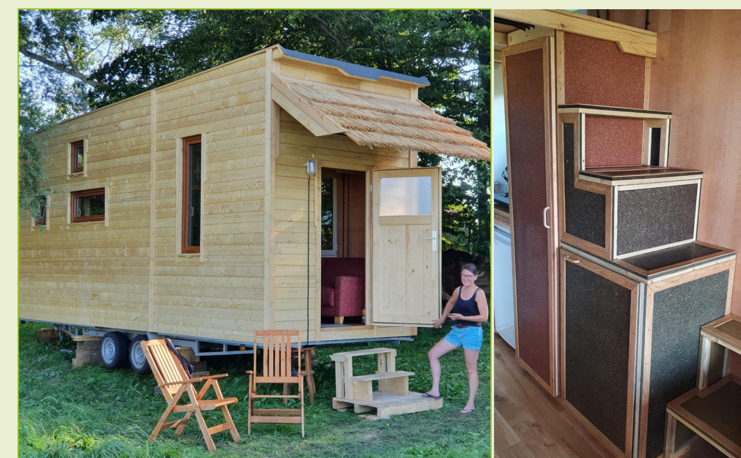
Fig. 1: left: Paludi-tiny house with thatched canopy, based on steel trailer; right: coloured furniture fibre boards made from wet meadow grass, reed and hemp.
