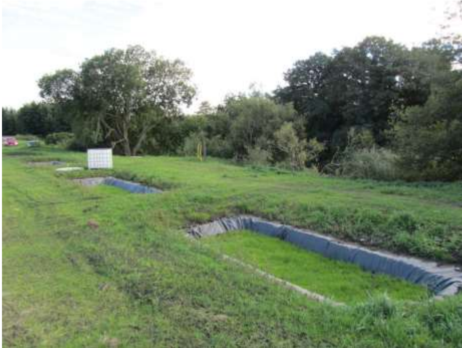
Figures: Constructed wetlands for the treatment of waters from agricultural catchment areas
